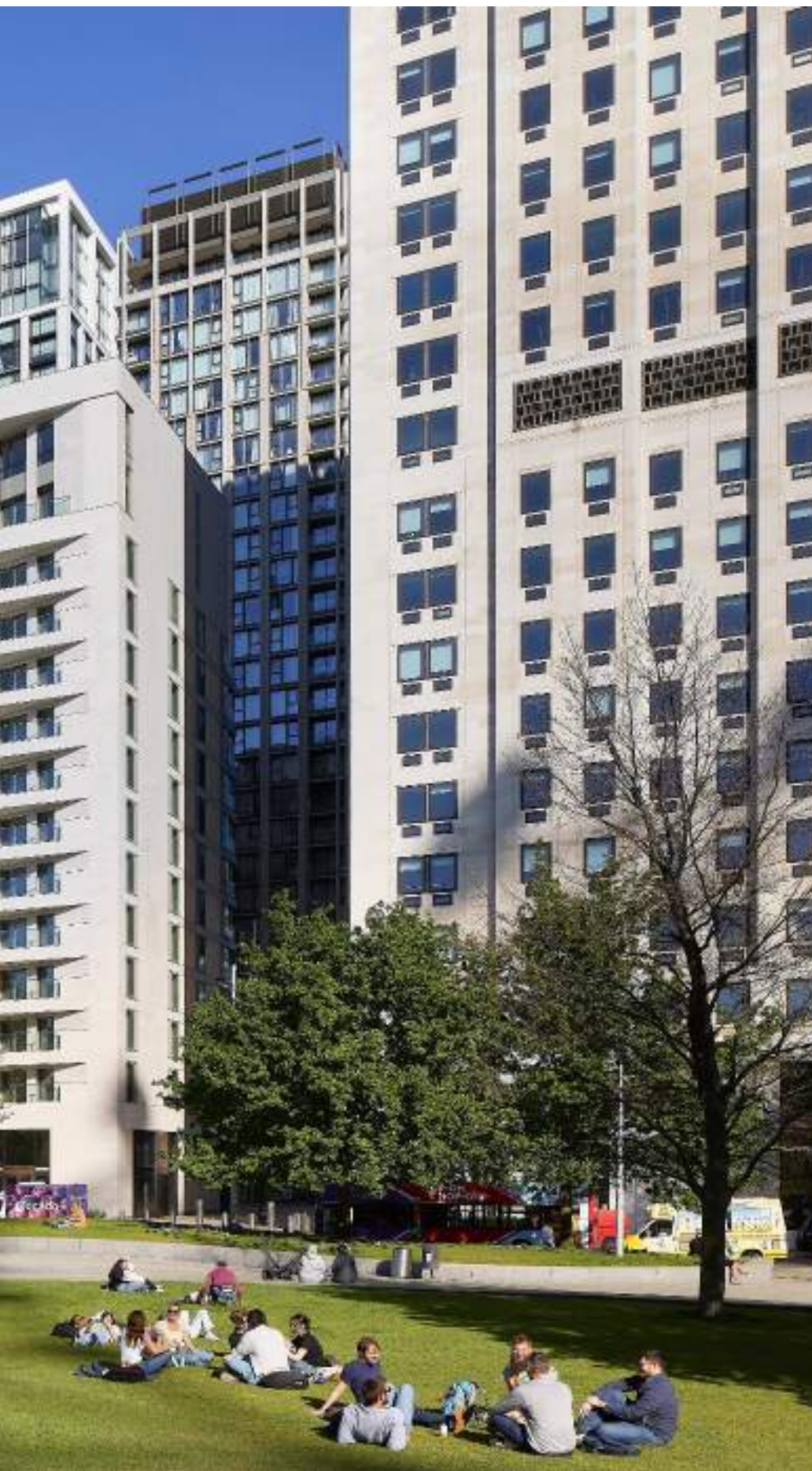
Left: Timeless and restrained, the building's limestone façade forms a dignified backdrop to Jubilee Gardens.
