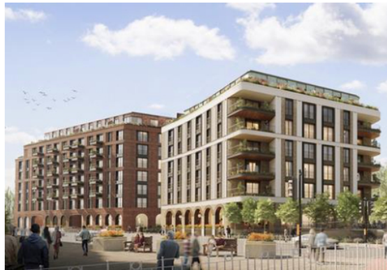
Plans to replace the Debenhams have been drawn up by Squire & Partners
