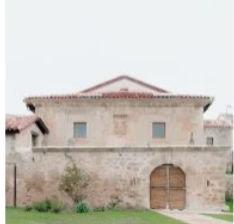
Stone ruins turned into Spanish holiday home by Atienza Maure Arquitectos
