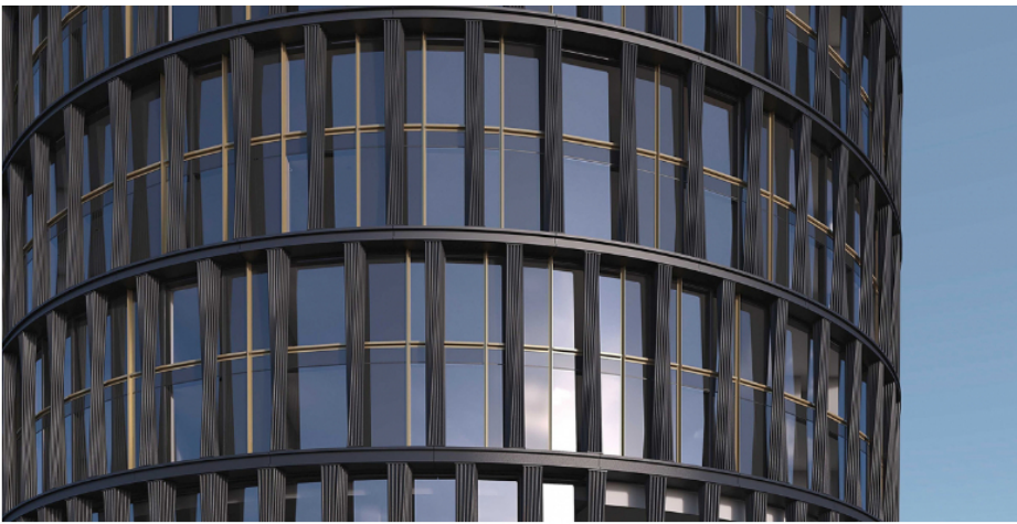
Each section of the cogwheel facade is extruded over two floors and articulated by a series of twisting metal fins.
