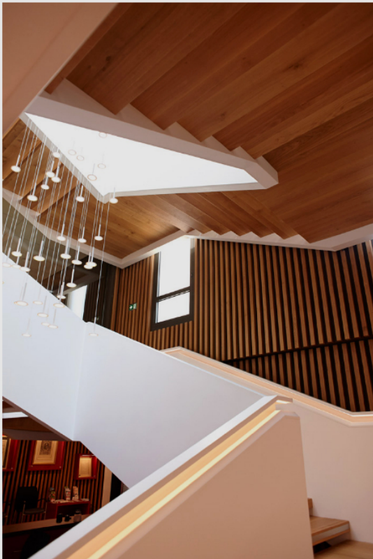
The atrium staircase is made of natural oak and HI-MACS
