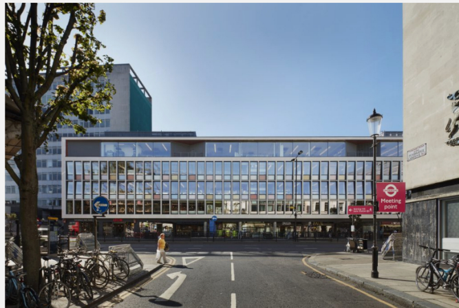
Refurbished South Block CREDIT: MATT CLAYTON
