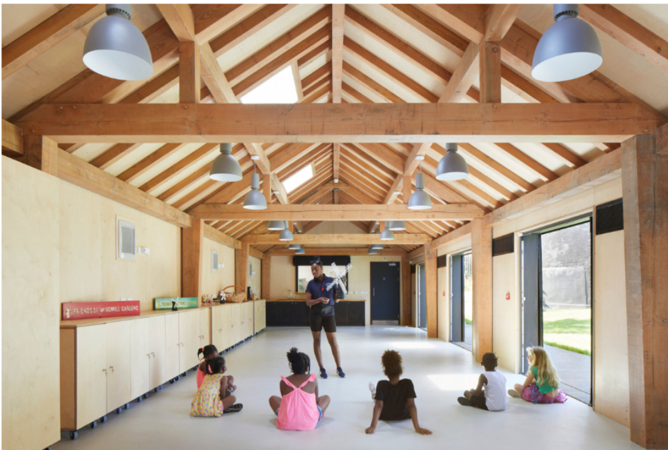
The building has a timber frame
