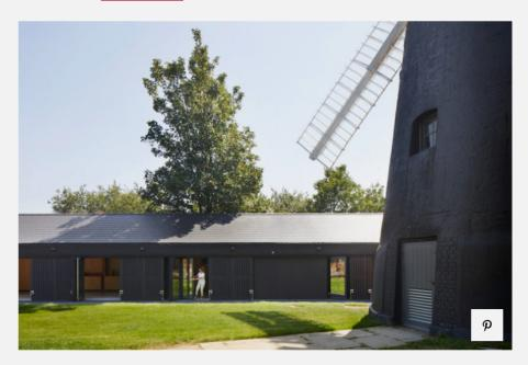
The bureau has built a modest, elongated one-story building that does not compete with the old mill. The design of the building was inspired by the historical buildings that stood on this site until the 1960s. The frame is made of Douglas fir, and the gable roof is made of Staffordshire blue engineered bricks, reminiscent of a pitch-black painted windmill tower.
