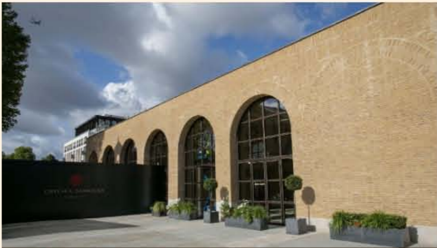
Bold brick arches and vaults impart a sense of permanence
