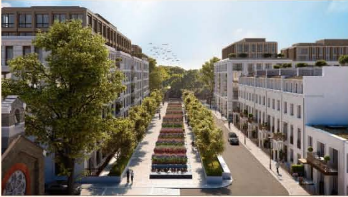
The new buildings are not attempting to create new typologies
