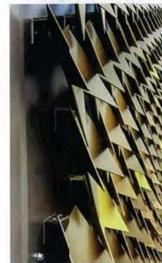
Above View through the living space to the roof terrace. Far left and right The metal-clad façade, inspired by nearby Virginia creepers, is inset with Schueco window systems. Left Shingle detail.
