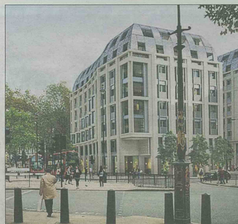
West Enders: developer Berkeley Homes is converting 190 Strand, a modern office scheme – as well as office blocks on the Albert Embankment – into homes
