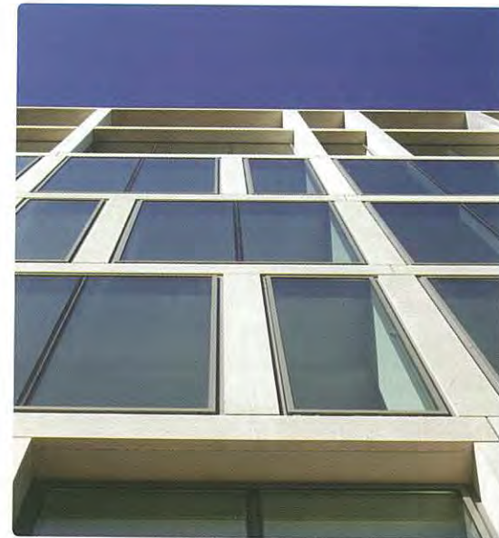
Flush and recessed glazing set within slender concrete columns.
