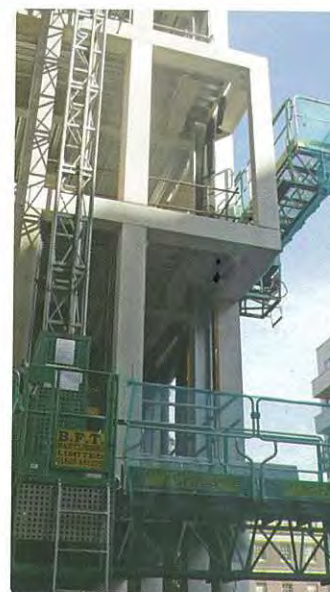
Installation of precast units.
