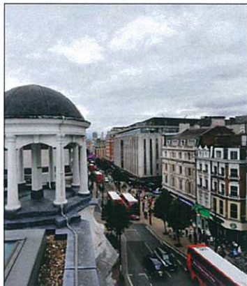
£1.65 million: 10 new apartments looking down over Oxford Street and New Bond Street are being built at Verge Mayfair (020 7861 5489)
