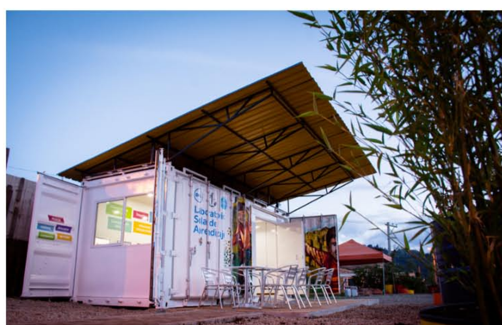
the zubabox is a solar-powered learning lab constructed from a recycled shipping container
