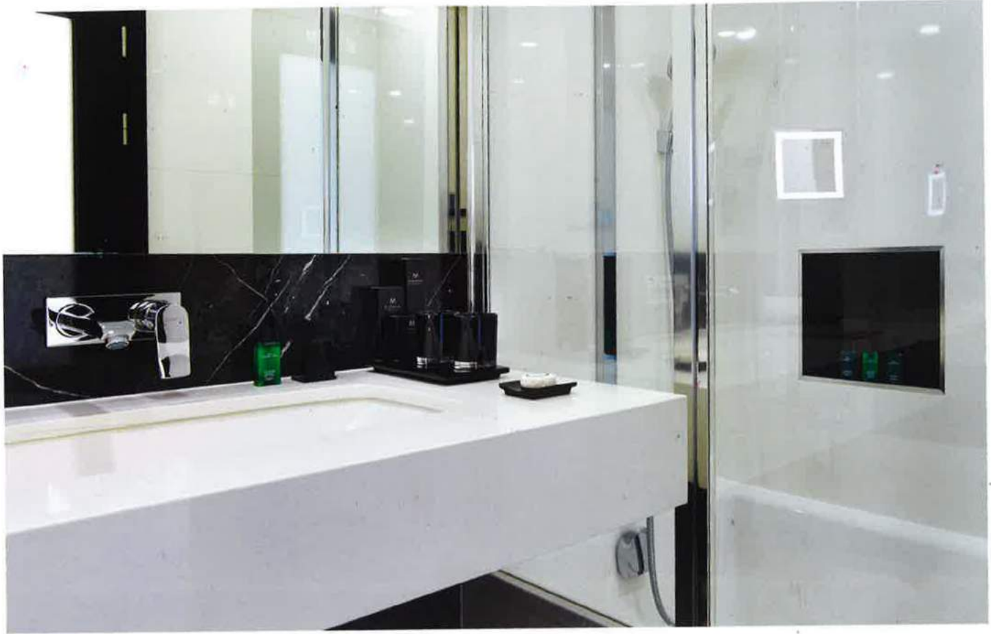
Above: Bathrooms have been fitted with Vitra M-Line basins and WCs by German design studio NOA, with fixtures by Hansgrohe
