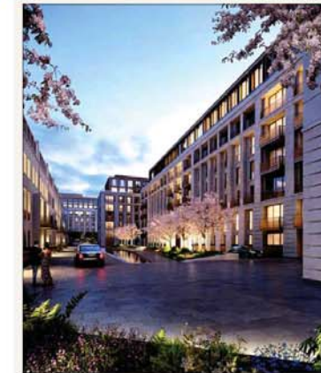
Super-prime: how the first phase of the Chelsea Barracks plan will look
