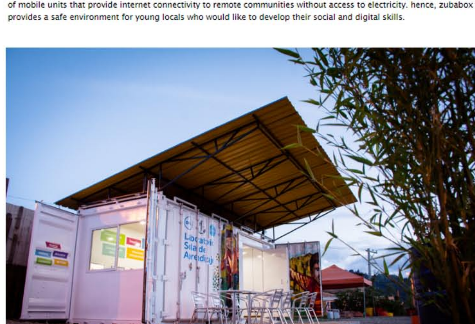
the zubabox is a solar-powered learning lab constructed from a recycled shipping container
