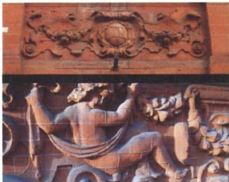
Top Facade and brickwork details.
