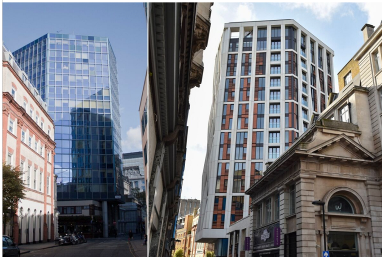
The Hexagon Apartments at Parker Tower, before (left) and after conversion. A second exterior was added to improve shade and cooling. Source: Squire and Partners, Photographer: John Keeble/Getty Images Europe
