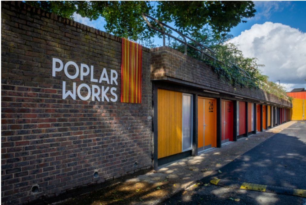
Empty garages on a housing estate were converted to workspace to create The Trampery's Poplar Works (PIC The Trampery)
